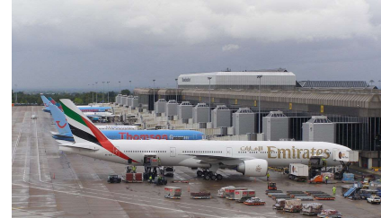
Manchester Airport Terminal 2 SBT Architects
