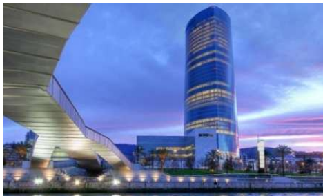
Tour Iberdrola – Bilbao Cesar Pelli & associates
