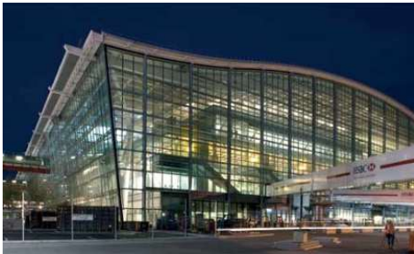
Heathrow Airport T2A – Londres Forster + Partners architects
